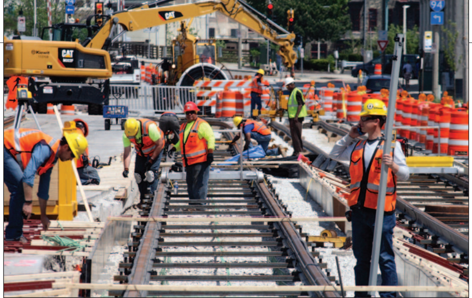
▲ On May 18, 2017, construction was underway on St. Paul Street. We are looking east from Second Street toward Plankinton Avenue.
