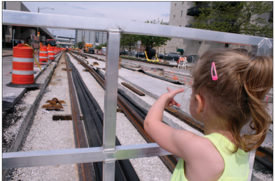
▲ Further west on St. Paul Avenue construction progressed enough that it was starting to resemble a streetcar Line. Gracie, then 2-½ years old, was visiting Grandpa who took her along on May 22, 2017. Standing on one of the pedestrian bridges to walk over the construction, Gracie pointed to the westbound track and said "train." In September 2018 Gracie and Grandpa attended the press conference at the car barn when Milwaukee Mayor Tom Barrett was announcing opening day. Every time the mayor said "Hop," Gracie would hop. Noticing this, Mayor Barrett called Gracie up to the podium to hop every time he said "Hop." She appeared in all the television newscasts that evening.
